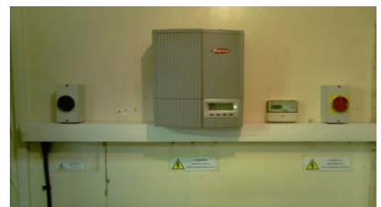
Solar DC/AC Inverter Layout
